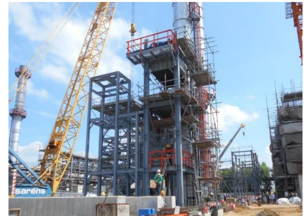
Boiler Stack/ Structure
